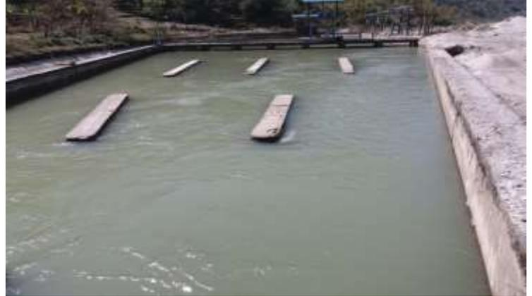
*Fig: Settling basin showing baffle wall*
