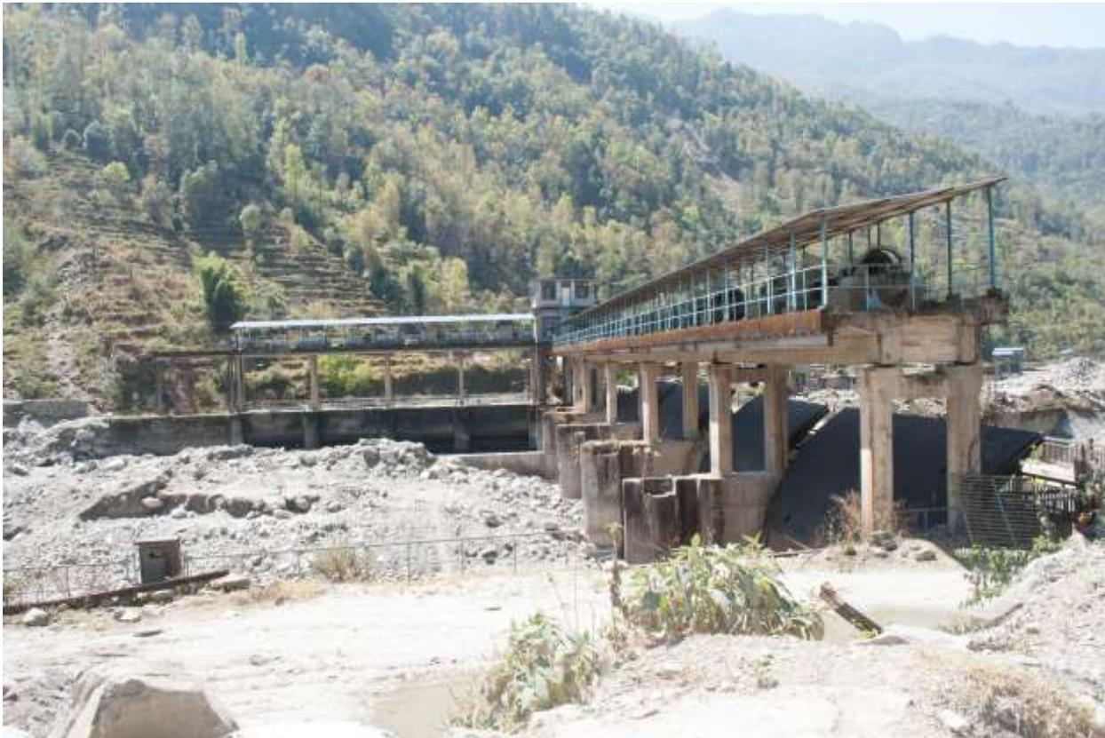
*Fig: Dam showing radial gates with hoist and intake*
