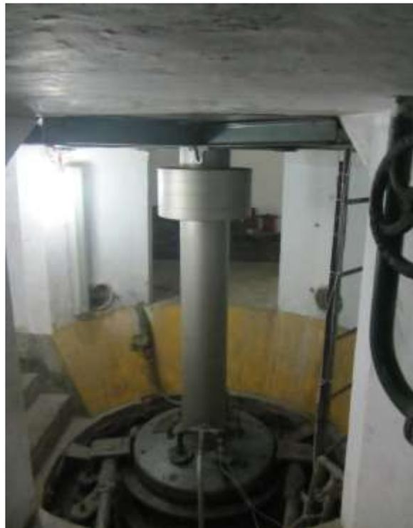
*Fig: Shaft of Turbine*
