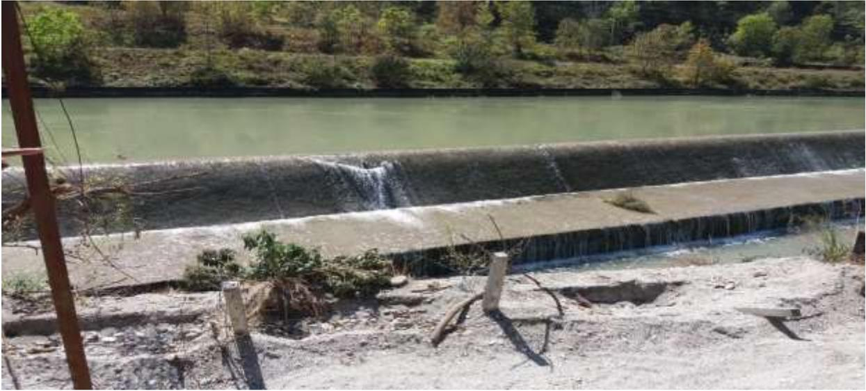
*Fig: Fore-bay with spillway*
