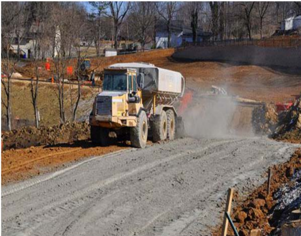
Fig: Soil Cement Stabilization
