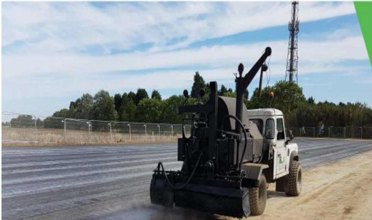
Fig: Bituminous Stabilization
