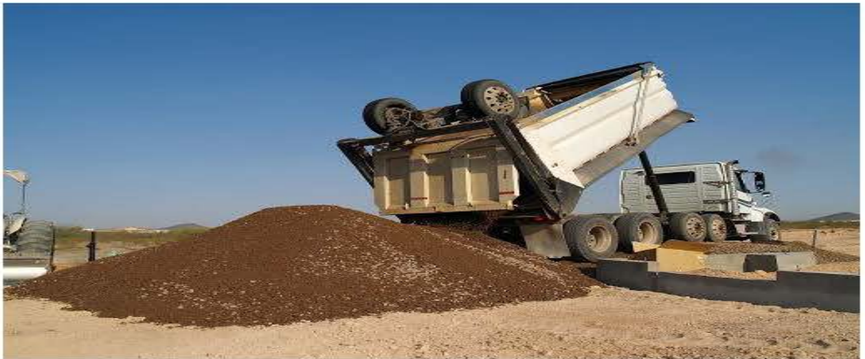
Fig: Mixing various sized aggregate for mechanical stabilization
