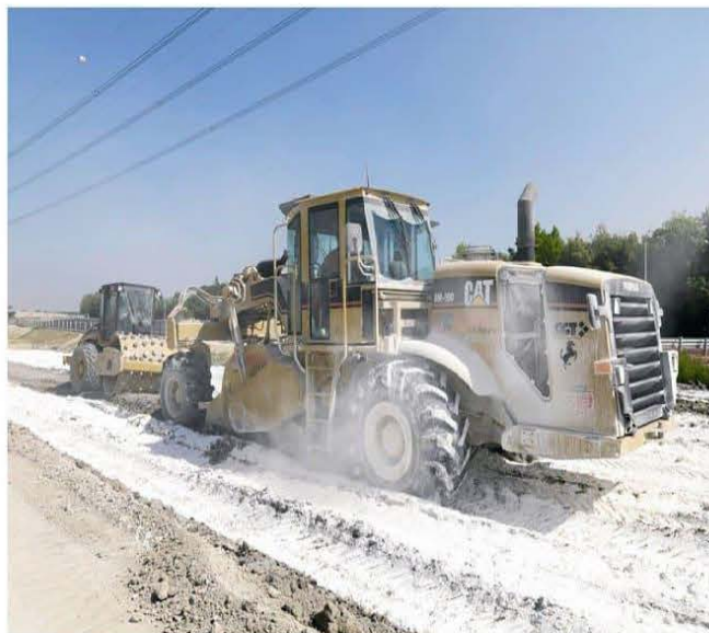
Fig: Soil Lime Stabilization
